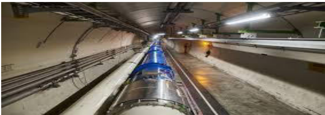
Figure 5.1 LHC Tunnel of CERN
